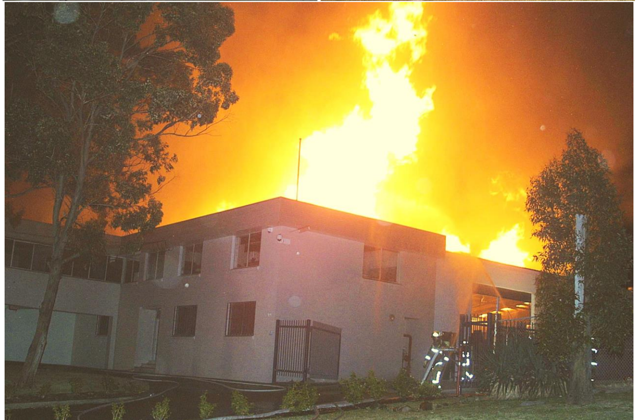
Flames at least 20 metres in height from the burning pallet stack vent into the night sky. Large flames roll across the roof of Exposure D factory, melting the roof skylights, allowing embers to enter. The factory wall has collapsed and firefighters are setting up a ground monitor to stop fire entering the factory.
