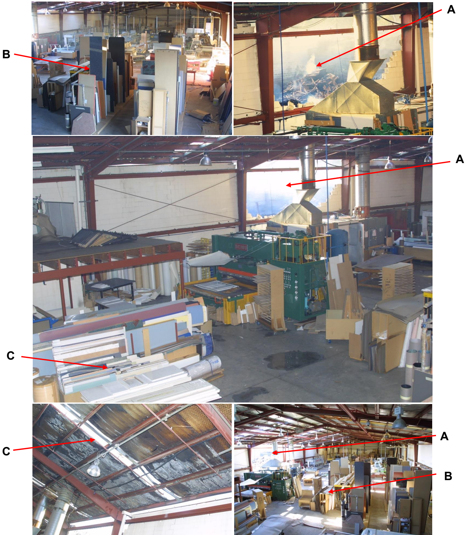
Exposure D: Fire intensity caused (A) a large section of the western wall to collapse, allowing fire to enter factory. Firefighters fought a determined battle to stop the fire spreading into the exposure, which contained (B) large quantities of combustible materials. Intense radiant heat also caused the (C) roof skylights to melt, creating large openings that allowed embers to enter the factory. Due to the efforts of firefighters, the factory was saved.
