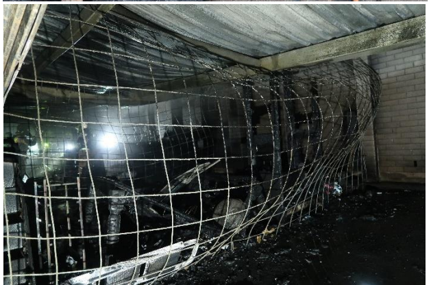
Garage contents consisted of a large variety of stored materials, representing a “witches brew” fuel load. Although some garages were lightly loaded, others were filled to capacity. Many contained hazardous materials including flammable liquids, LPG cylinders and aerosols.
