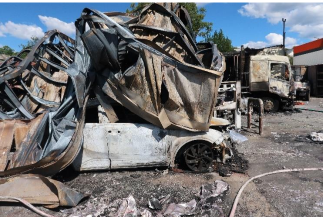
Significant damage occurred to the petrol tanker, several motor vehicles, fuel pumps, the service station building and overhead steel awning due to the fire intensity.
