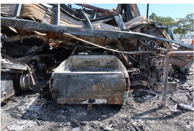
Significant damage occurred to the petrol tanker, several motor vehicles, fuel pumps, the service station building and overhead steel awning due to the fire intensity.
