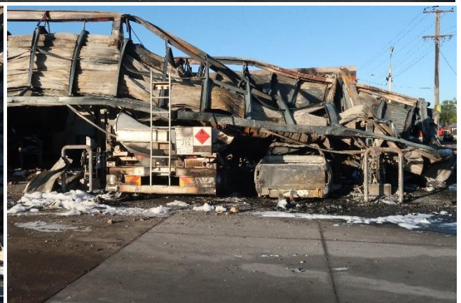
The tanker was parked beneath the service station awning when the fire broke out. Intense heat from the burning petroleum caused the structural steel supporting the awning to collapse. Steel roof sheets collapsed onto the tanker, acting as a barrier restricting firefighting streams from reaching the fire.
