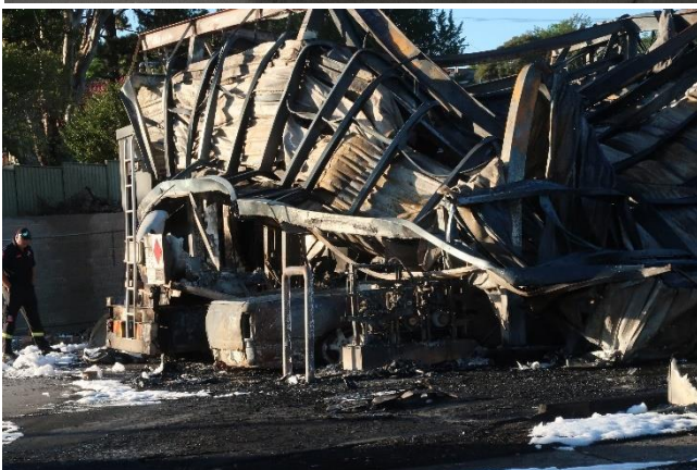
The tanker was parked beneath the service station awning when the fire broke out. Intense heat from the burning petroleum caused the structural steel supporting the awning to collapse. Steel roof sheets collapsed onto the tanker, acting as a barrier restricting firefighting streams from reaching the fire.
