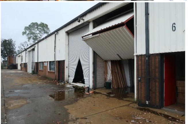
The main fire occupancy contained a second cool room (top left) and an office (top right). A combination of fire activity and hose streams resulted in some elevated stock becoming unstable and collapsing (middle). The factory units were fitted with two types of doors; steel roller shutter doors (lower left) and steel horizontal bi-folding doors (lower right).
