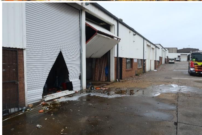
The main fire occupancy contained a second cool room (top left) and an office (top right). A combination of fire activity and hose streams resulted in some elevated stock becoming unstable and collapsing (middle). The factory units were fitted with two types of doors; steel roller shutter doors (lower left) and steel horizontal bi-folding doors (lower right).
